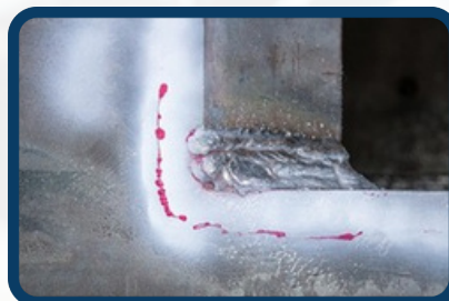
Penetrant Testing (PT):
