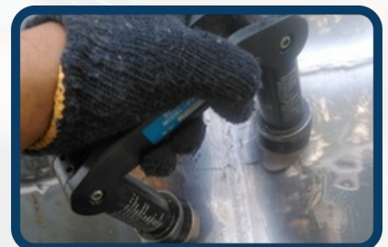
Magnetic Particle Testing (MT):
